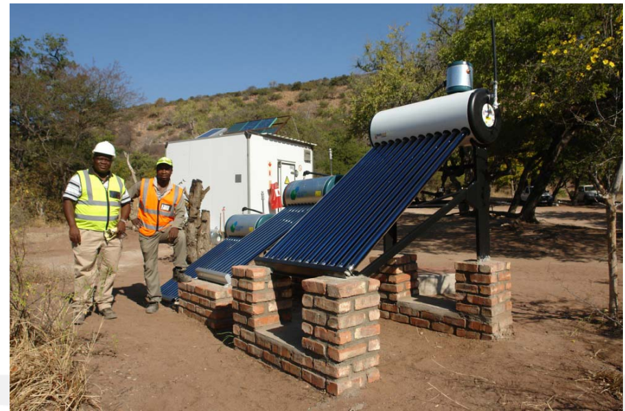
Tanga Camp - Recent installation of solar heating panels for hot water
