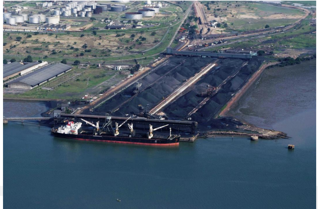
Matola dry bulk terminal
