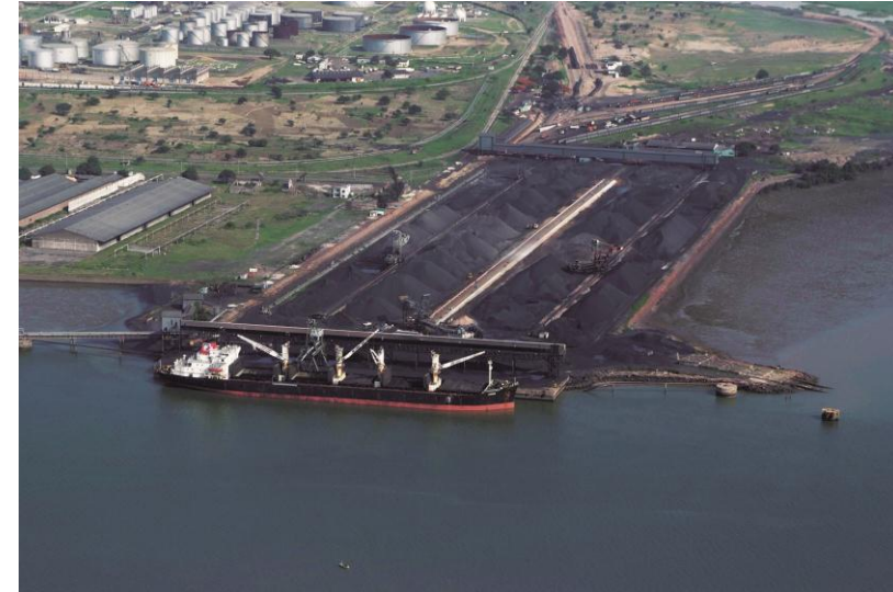
Matola Dry Bulk Terminal
